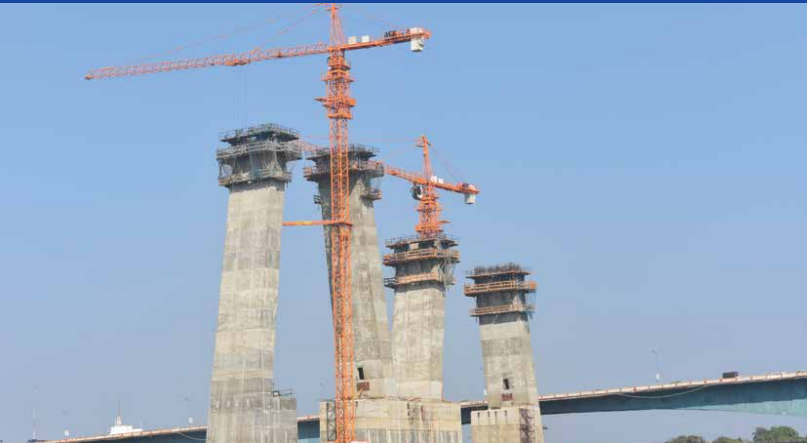
Zuari bridge, Goa
